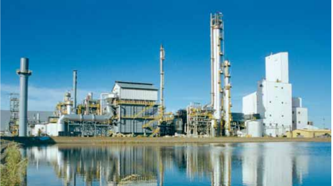
Ammonia and Urea plant Saskferco; Canada
